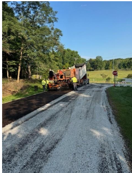
Motor paving layer on entry drive at O'Neil Woods Metro Park
